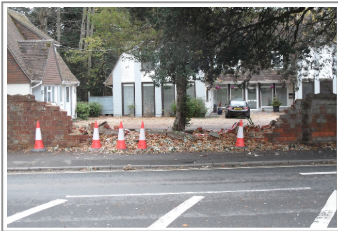
Photo 1: The demolished section of wall
