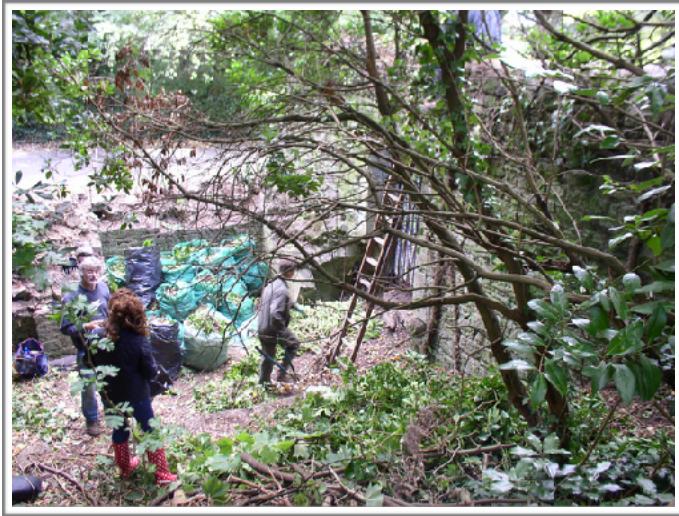
Photo 1: Clearing the Priory Walls in 2010
