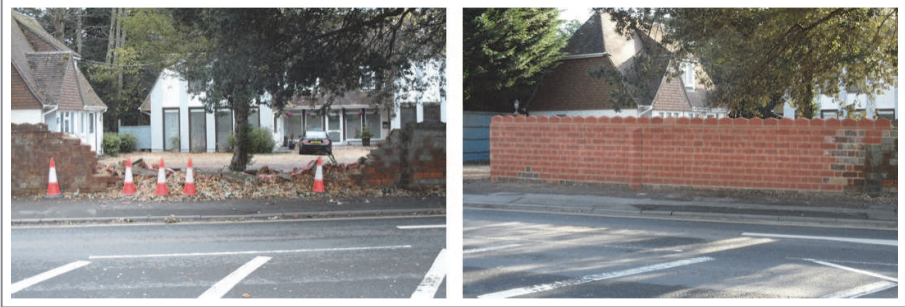
Left: The demolished wall; Right: The wall restored
