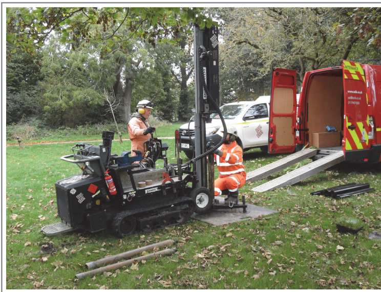
The Dando Terrier drilling rig being off-loaded at Druitt Gardens
